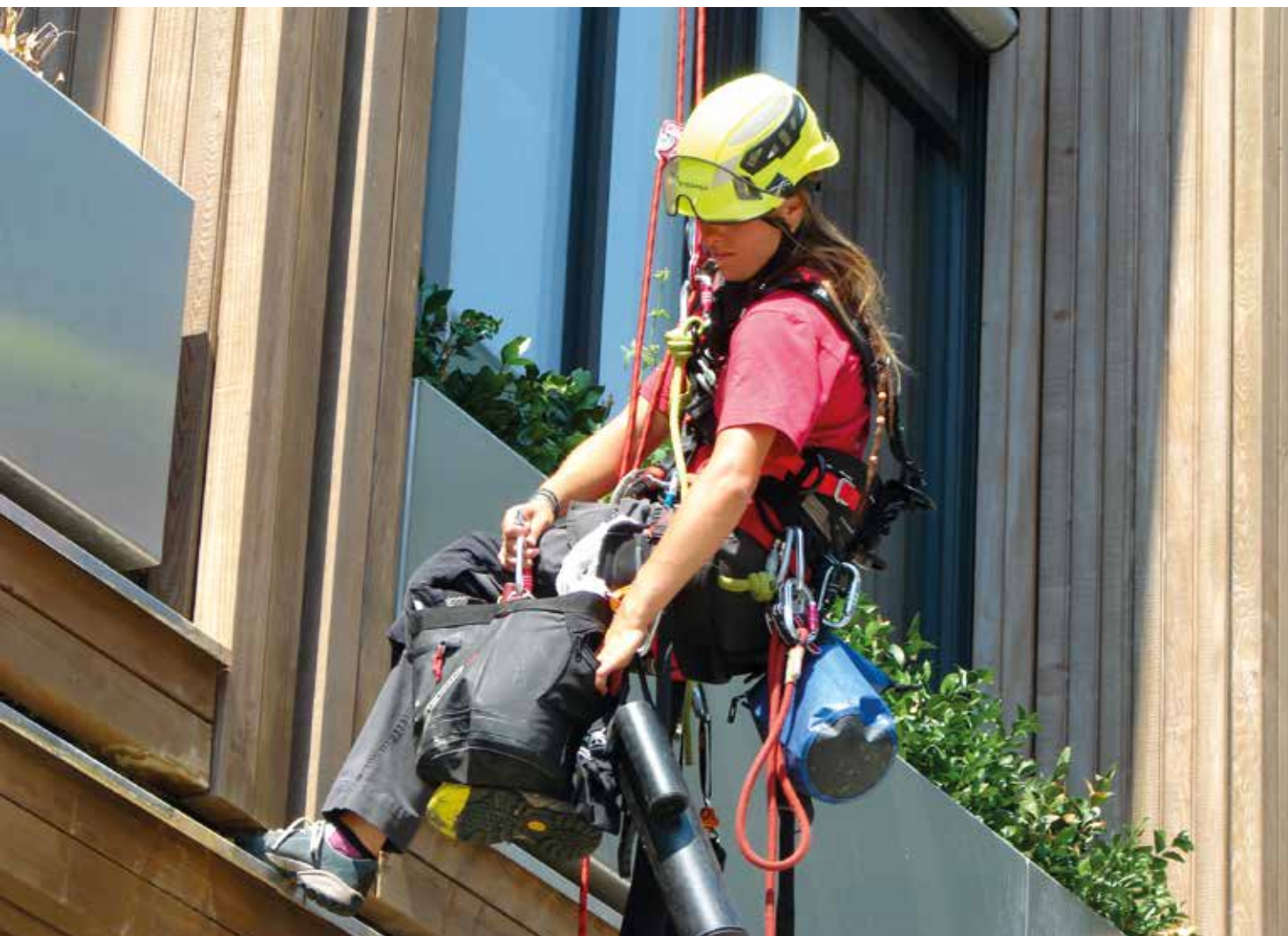
Gutter modification for a new building in Geneva (MSF). Modificación de los flujos de agua para el nuevo edificio en Ginebra (MSF). Genève, Switzerland (courtesy of Corde-Access SA, rigger Jenna Piron, ph. Corde-Access SA).
