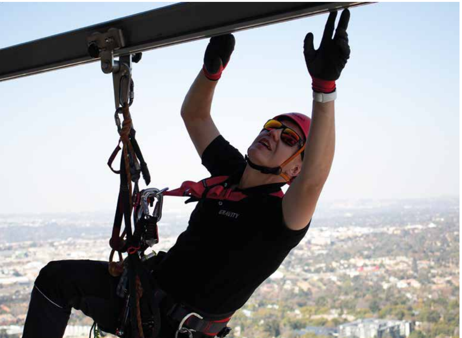
Martyn Cilliers doing maintenance operations on the Leonardo building, using C.A.M.P. gear and the Gravity Secuirail. Martyn Cilliers realiza el mantenimiento del edificio Leonardo, utilizando equipos C.A.M.P. combinados con Gravity Secuirail. Sandton, Johannesburg, South Africa (courtesy of Gravity Gear Pty Ltd, ph. Ethan de Witt).
