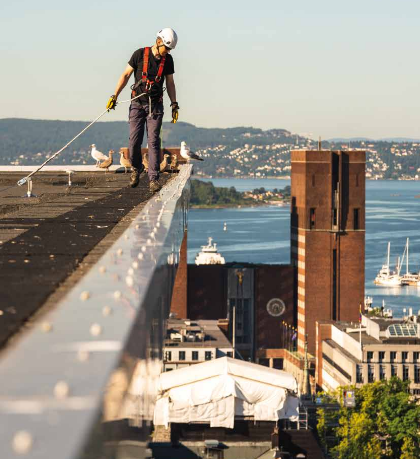
Torbjørn Solheim inspecting a roof with a beautiful view on the fjord. Torbjørn Solheim inspecciona un tejado con magnificas vistas del fiordo. Universitetsgata 2, Oslo, Norway (courtesy of Varri AS, ph.Kyrre Buxrud).
