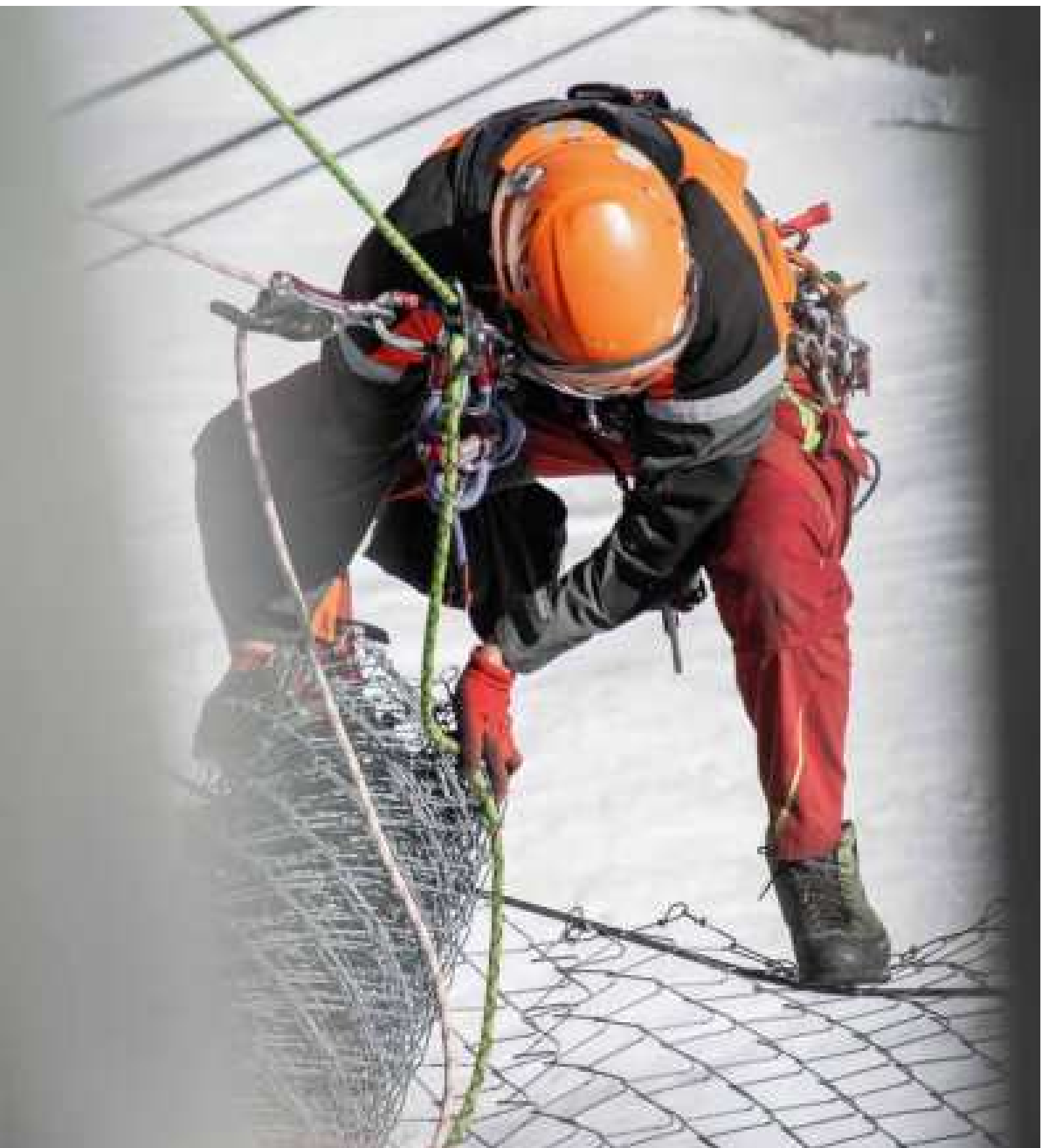
Installation of anchor points and safety nets for the reconstruction of the famous “La Botta” restaurant at Glacier 3000. Instalación de anclajes y redes para la reconstrucción del famoso restaurante «La Botta» en Glacier 3000. Les Diablerets, Switzerland (courtesy of Corde-Access SA, riggers Andrea Giuzzi & Julien Guisolan, ph. Ari Cretton).
